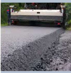
Paving thicknesses up to 300 mm.
