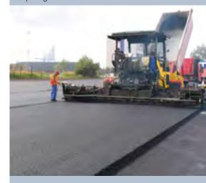
Fixed screeds for large width paving.
